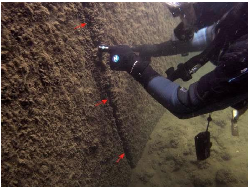
Figure 2: Technical inspection by Scientific Divers. Especially the in-situ documentation is crucial as an objective risk assessment is not possible from the water surface.
