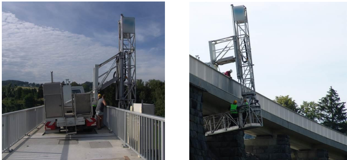
Figure 1: Technical inspection at high altitudes with an underbridge-inspection-unit.
